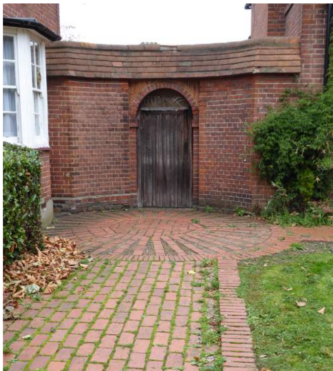
Original brick pavers
