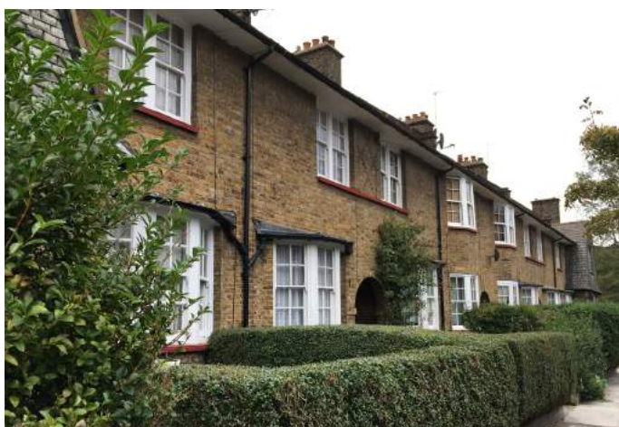
Tower Gardens Road (north side)
