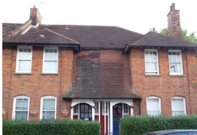
Shobden Road (porch cat slide roofs)
