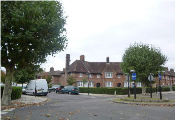
Junction of Risley Avenue and Awlfield Avenue
