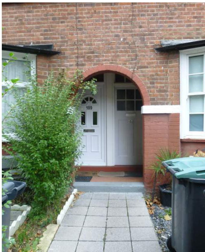
Replacement door (left) original door (right)
