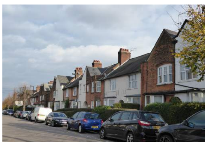
Painted brickwork disrupts cohesion of this terrace
