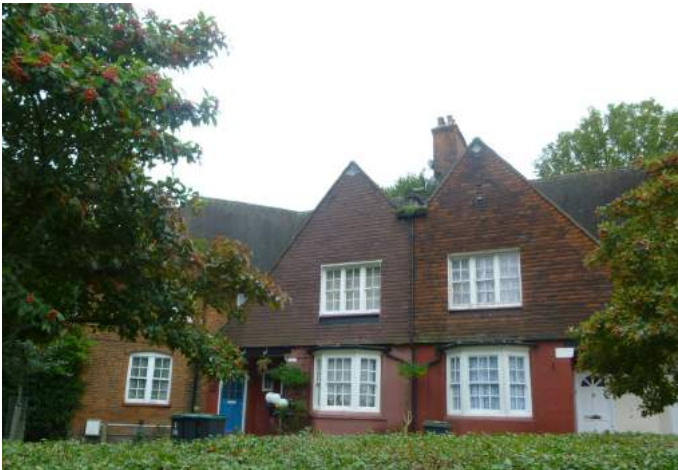
Junction of Risley Avenue and Awlfield Avenue
