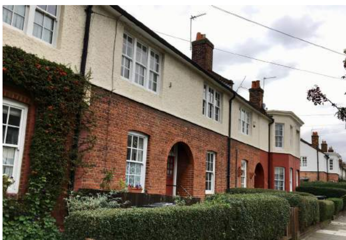
Tower Gardens Road (north side)
