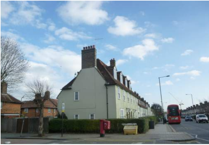
Lordship Lane: cottage flats
