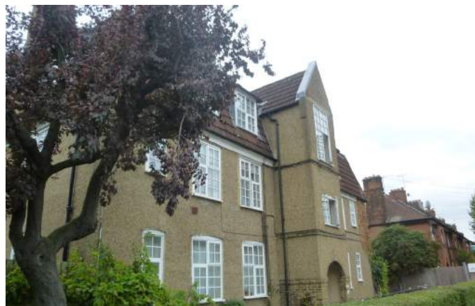
Topham Square: Risley Avenue elevation
