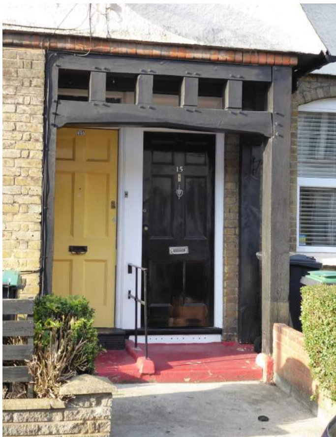
Seward Road porch detail
