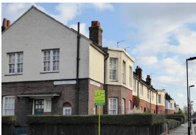
Tower Gardens Road (north side)
