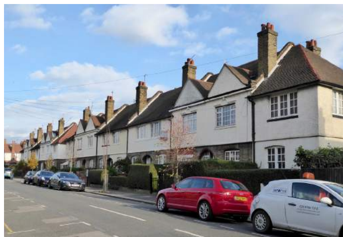
Teynton Road (east side)
