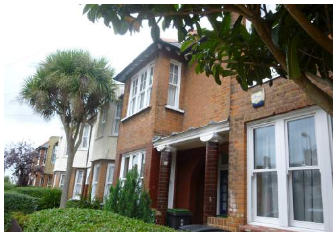
Tower Gardens Road (north side)
