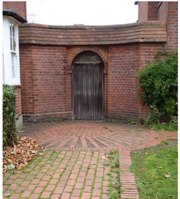
Original brick pavers
