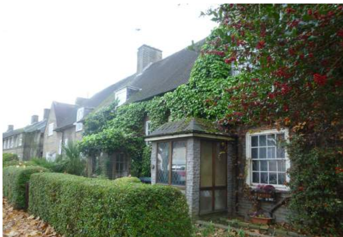
Modern porch additions
